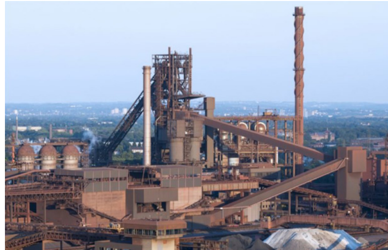
thyssenkrupp's plant in Duisburg's Schwelgern section (source: thyssenkrupp AT.PRO tec GmbH)
